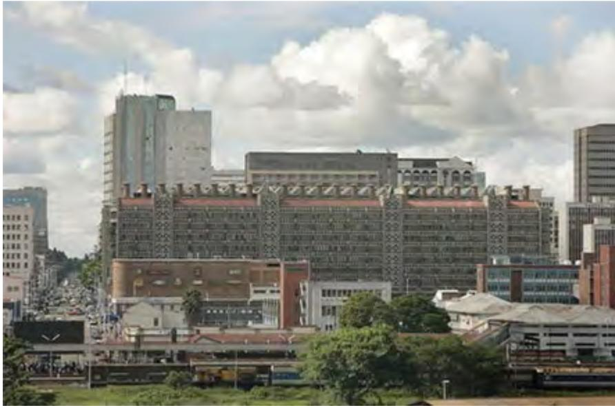
The Eastgate Centre is a shopping centre and office block in central Harare , Zimbabwe. The building was designed to be ventilated and cooled entirely by natural means — it was biomimetically modeled on local termite mounds. It was probably the first building in the world to use natural cooling to this level of sophistication.
